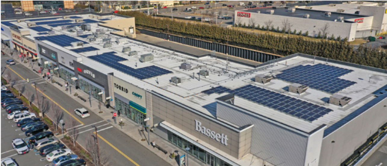
Chimney Rock Solar Panels
