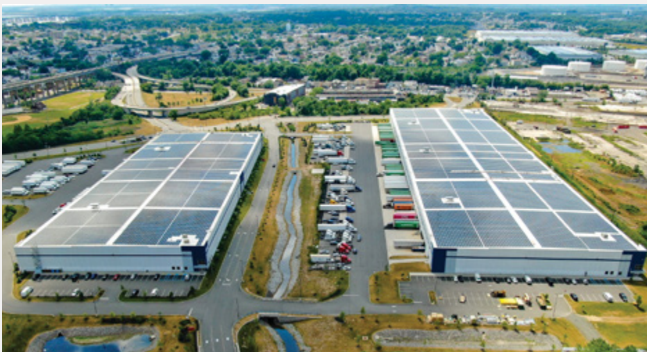
Perth Amboy, New Jersey Community Solar Panels
