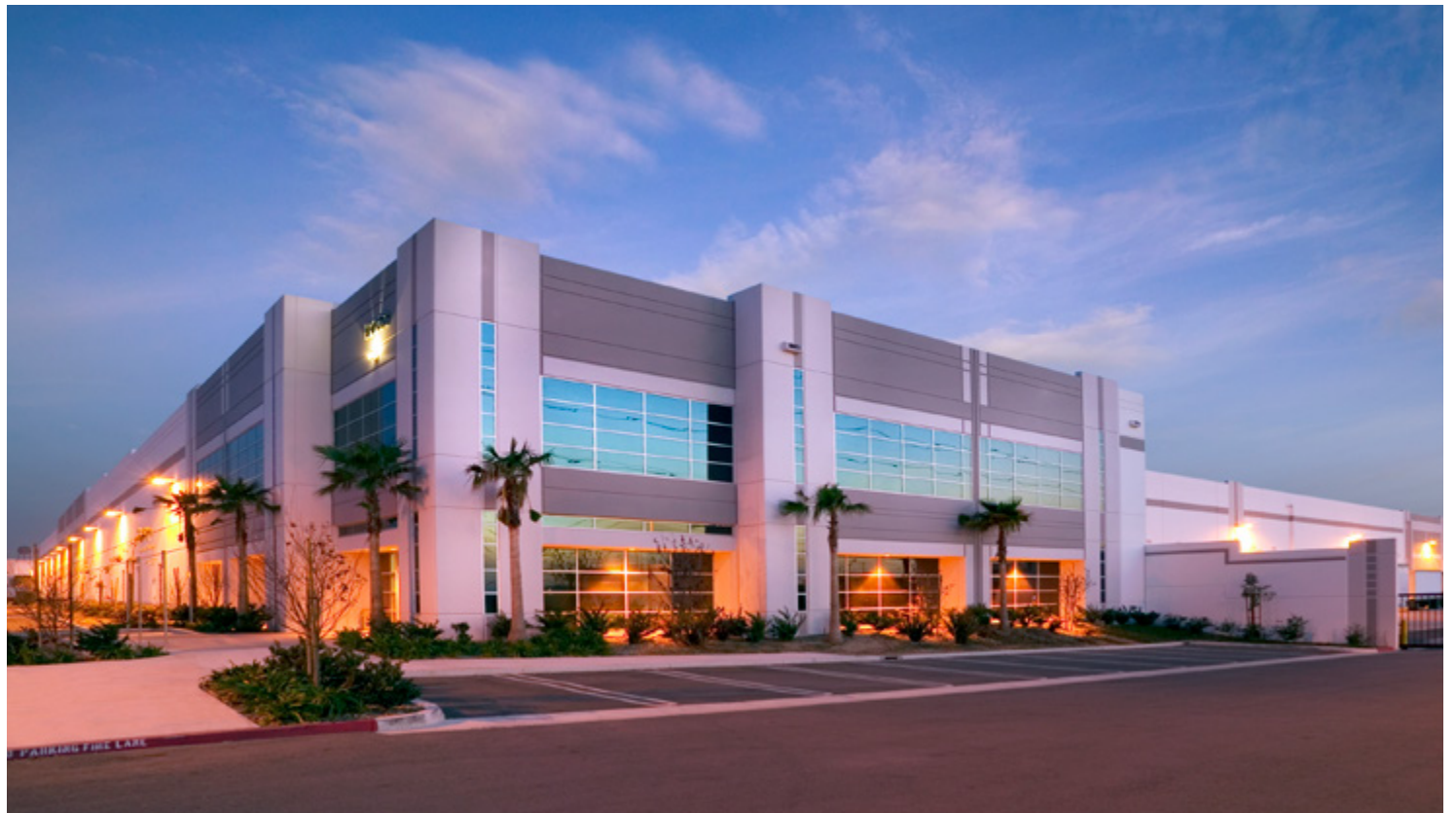
Prologis, Inc., Kaiser Distribution Center, Fontana, CA
