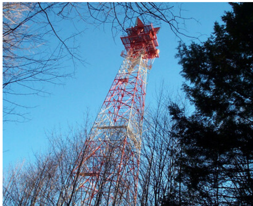
American Towers, Blood Hill Road Tower, Windsor, VT
