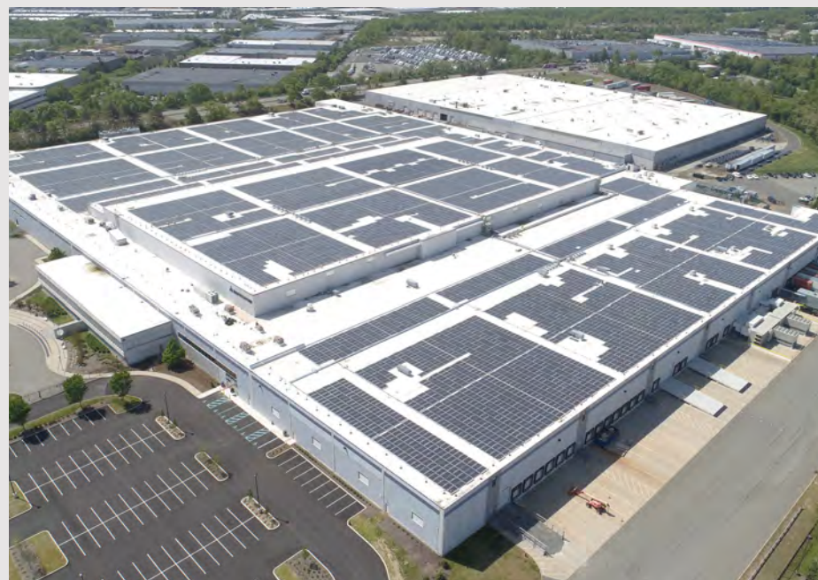
New Jersey data center rooftop solar array
