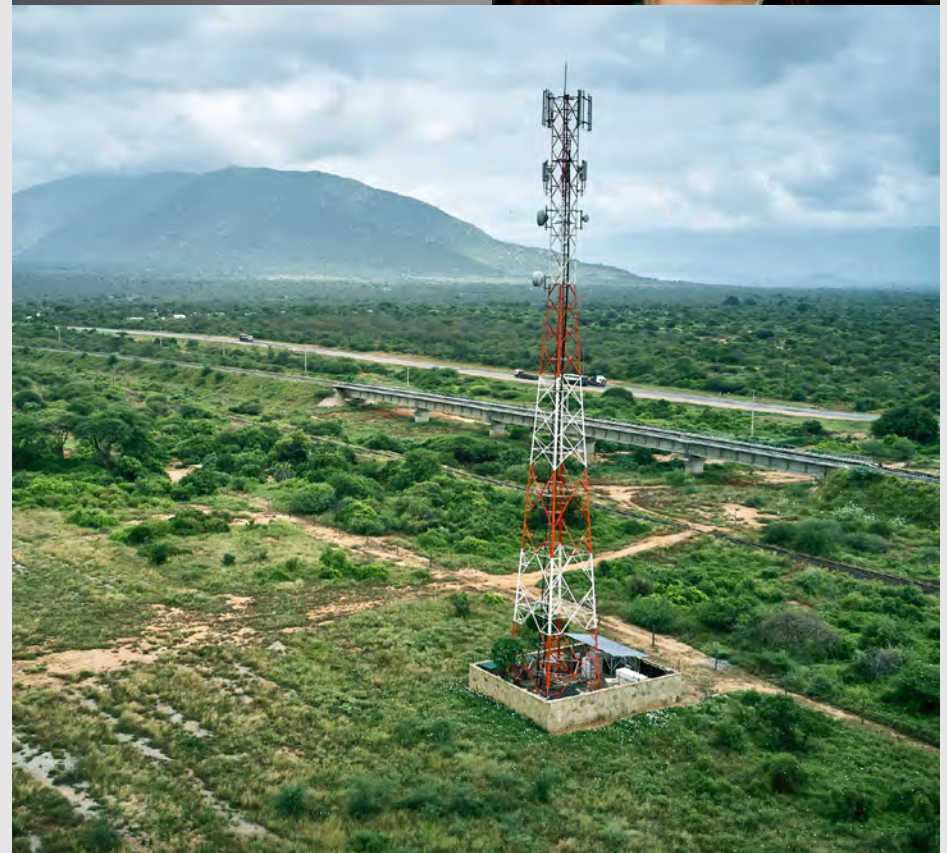
Self-support tower in Kenani, Kenya with on-site solar photovoltaic power generation.
