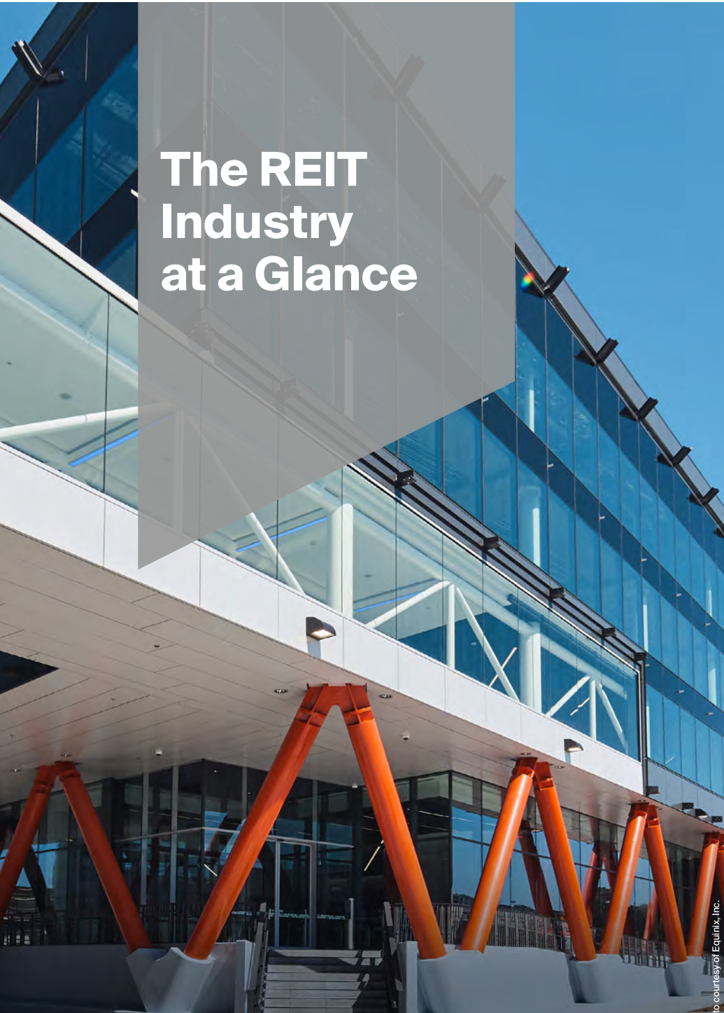
Exterior of Equinix SV5 International Business Exchange™ (IBX®) in Singapore
