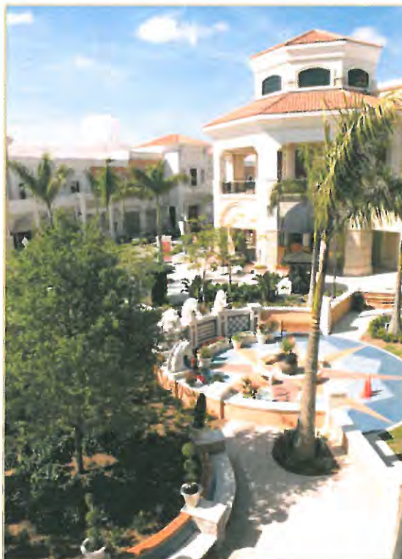
The 511,000-square-foot Village at Gulfstream Park is an open-air lifestyle center in Hallandale Beach, Florida, featuring dining and retail, and anchored by Gulfstream Park racetrack.
